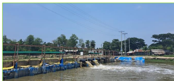
Kalishakul (Bhobodoho), Avaynagar, Jashore
